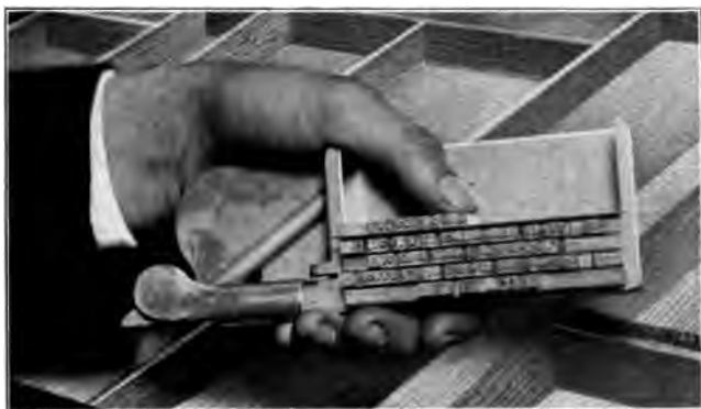
FIG. 10. Showing correct method of holding stick
